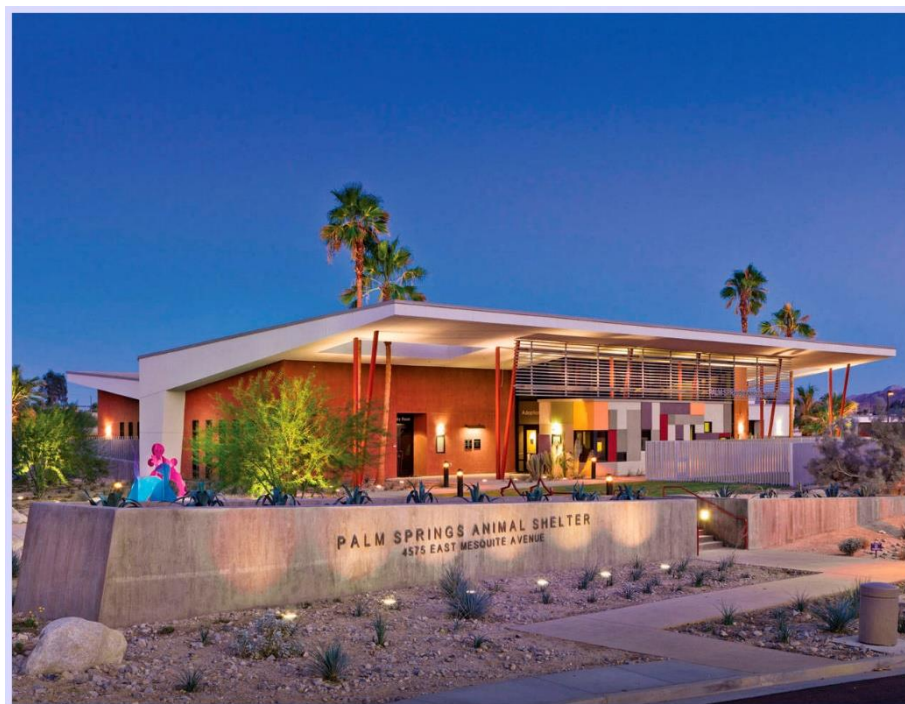
Figura 20: fachada do projeto Palm Springs Animal Care Facility.
