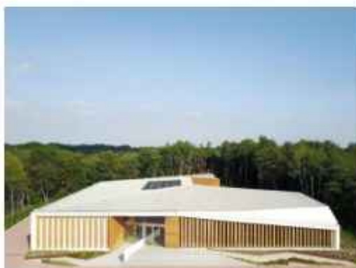
Figura 2 - Restaurante Wood Court – vista externa (FONTE: ARCHDAILY 2020)
