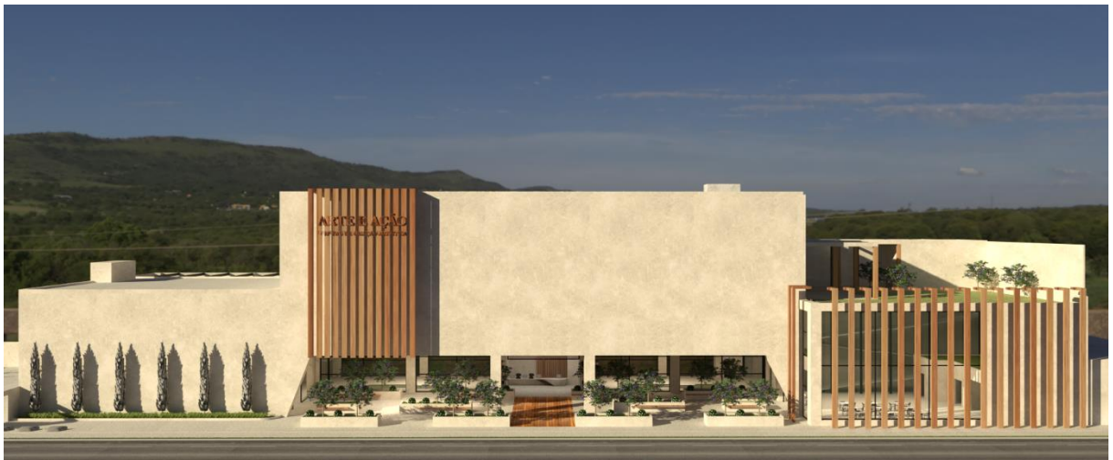
Figura 65 – Fachada principal / Final.
